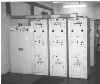
The next equipment changes came with SSB. The old DSB only W5 and the Mercury receivers were no longer suitable, so along came single frequency Ajax transmitters feeding through a combiner unit to a wideband aerial and Eddystone EC958 receivers.
