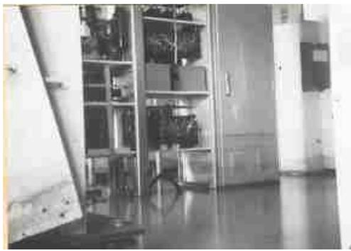
The same transmitters were brought back in to service, but this 'tide level mark' on the W5 could be seen throughout the rest of its service. I know – during maintenance periods I tried without success clean it off.
