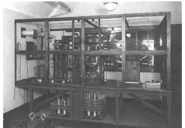
The Main receiver was a Marconi Type 12A direction finding receiver used for the main 600-metre band.
